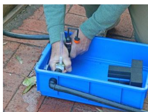
Float shaft must be vertical
