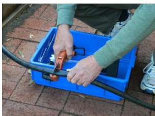
Cut the water supply pipe
